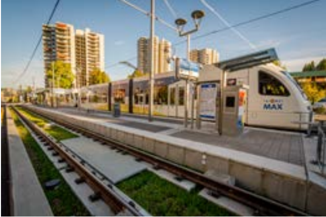
Eco-track at Lincoln St/SW 3rd Ave MAX Station.
