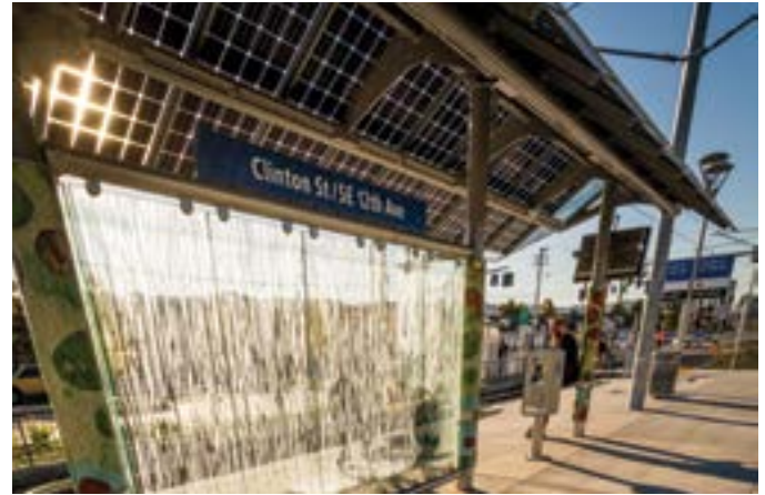
Solar panels on a Clinton St/SE 12th Ave MAX station platform.
