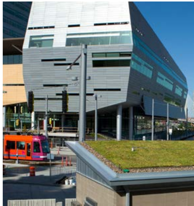
Eco-roofs help lower urban air temperatures.
