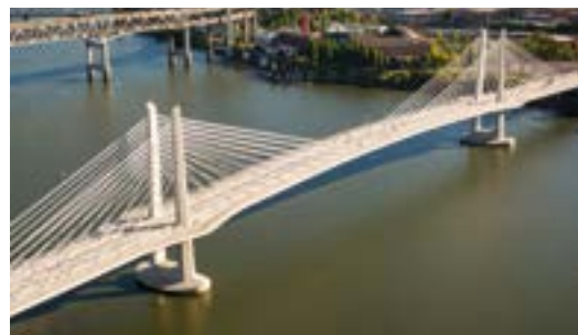
Tilikum Crossing is a 1,720-foot-long structure.
